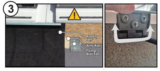
Cut the roofing around the hinge. Silicone between the hinge and roofing membrane.
