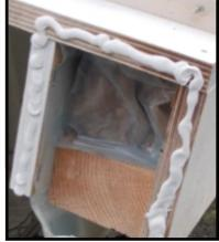
**4.** Apply white silicone on both sides of upstand as shown in above image.
