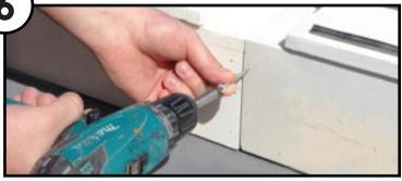
6. Fix into place using 2 screws (on right hand side - female upstand)
