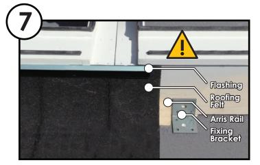
7. Fix upstand to roof with fixing brackets. Arris rail can now be fixed around bottom of the upstand. Roofing membrane can then be applied to upstand and flashing fitted.
