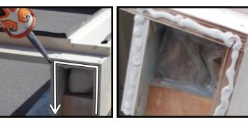
3. Apply white silicone on both sides of upstand as shown in above image.
