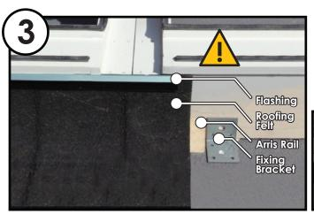
3. Fix upstand to roof with fixing brackets. Arris rail can now be fixed around bottom of the upstand. Roofing membrane can then be applied to upstand and flashing fitted.
